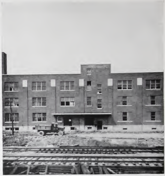
Carl Hansen Laboratory, West Allis, Wisconsin W. H. Buemming, Arch., Milwaukee, Wis. Osthoff & Peterson, Engrs., Milwaukee W. W. Oeflein, Inc., Contractor, Milwaukee, Wis. Tews Lime & Cement Co., Dealers, Milwaukee, Wis. Medusa Waterproofed Gray Portland Cement used.
